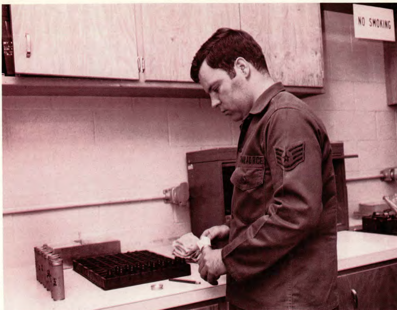
Accuracy is vital to the NDI Program. When taking oil samples, mark the sample bottle with the engine's identification, fill out the oil analysis request, and place both in the marked container before taking other samples. Lab people must be just as careful when analyzing the oil.
